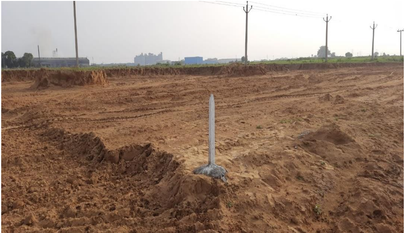
Bhiwadi Unit II Site Picture
