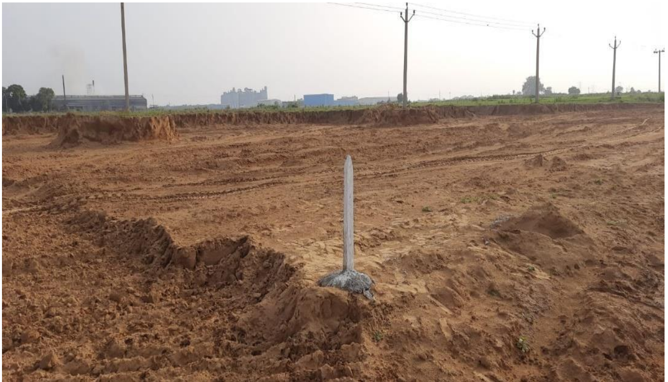
Bhiwadi Unit II Site Picture
